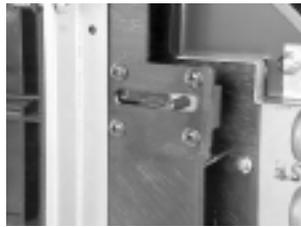
An open vent door brings unconditioned outdoor air into the room, increasing heating and cooling costs.
