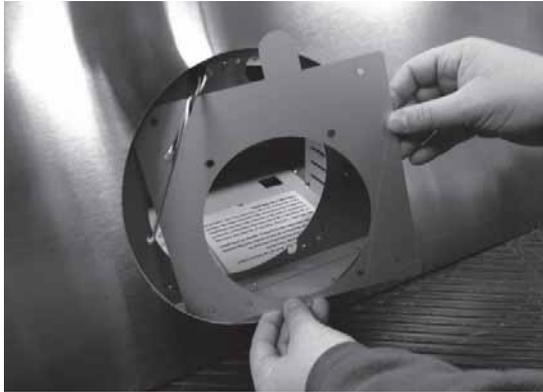
1. Remove internal blower flange plate.
