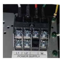
The outdoor unit is powered by 208/230 volt single phase electricity connected at the terminal block.
