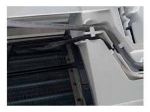
The Ambient (room) Temperature Sensor is a negative coefficient thermistor that will decrease in resistance with increases in room air temperature. The sensor is located on a clip mounted in the return air stream.
