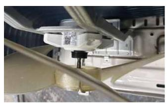
The fan motor is a variable speed motor. The required speed is calculated by the PCB. The motor is electrically connected to the PCB via PLUG CN- 10
