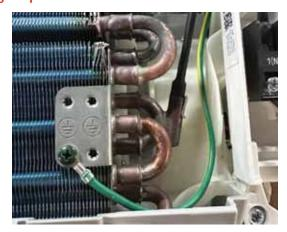
The Piping Temperature Sensor is a negative coefficient thermistor that will decrease in resistance with increases in coil temperature. The sensor is located in a socket soldered to the surface of the indoor coil.
