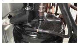
The Discharge Temperature Sensor is a negative coefficient thermistor that senses the temperature of the compressor hot gas. The PCB monitors the temperature of the compressor hot gas and will make inverter speed changes in response to input from this device.
