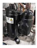
The compressor is a three phase DC inverter driven rotary type, capable of variable speed operation. The compressor operating frequency will be determined by the temperature difference between set point and room temperature.
