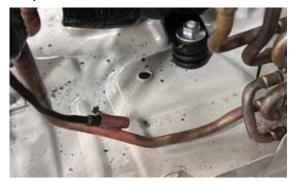
The Defrost Temperature Sensor is a negative coefficient thermistor that will change resistance in response to outdoor coil temperature changes. The PCB monitors the temperature of the outdoor coil to determine when the system should perform a defrost cycle. The sensor also monitors coil temperature during defrost cycles to determine termination conditions.
