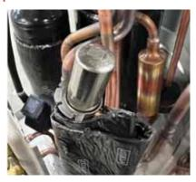
The metering device is an electronic expansion valve. The valve consists of an electrical operator and a valve body with internal variable size orifice. When operating, the PCB will send pulses of voltage to the electrical operator. The operator will then magnetically move the position of the metering orifice pin to vary refrigerant flow.
