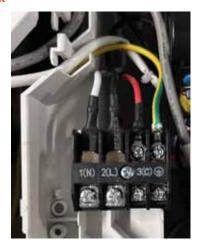
The unit terminal block receives electrical power from the outdoor unit. There are 4 connections for electrical wires. Terminals 1 and 2 are connected to terminals 1 and 2 of the outdoor unit. This wiring supplies power to the indoor unit.
