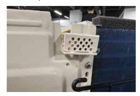
The Ambient Temperature Sensor is a negative coefficient thermistor that will change resistance in response to outdoor air temperature changes. The PCB monitors the temperature of the outdoor air to determine fan speed requirements and inverter speed. The sensor also plays a role in calculation of required defrost conditions.
