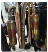
The system has debris-catching strainers that protect internal system components from contaminants in the refrigerant. The strainer is a permanent part that is not typically replaced.
