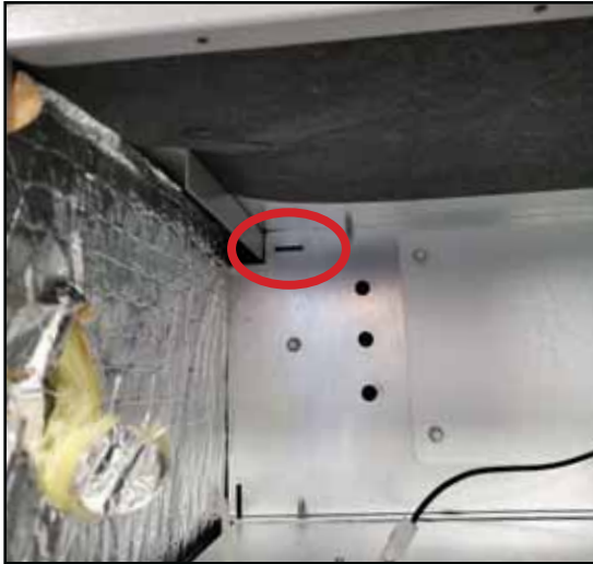
Figure 12. Notch for Control Panel Relocation
